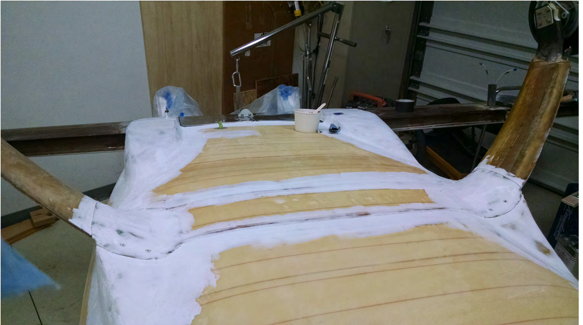
Fill around gear closeout and strakes. October 2017
